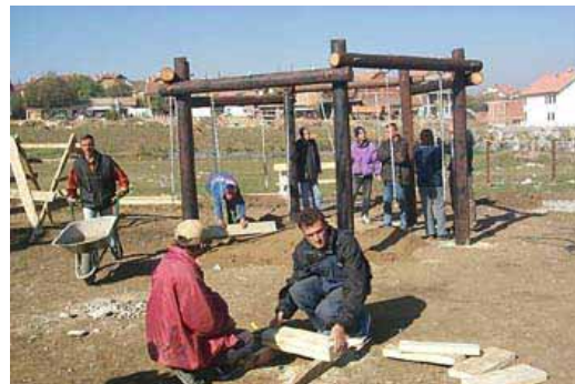
Playground swings being constructed.
