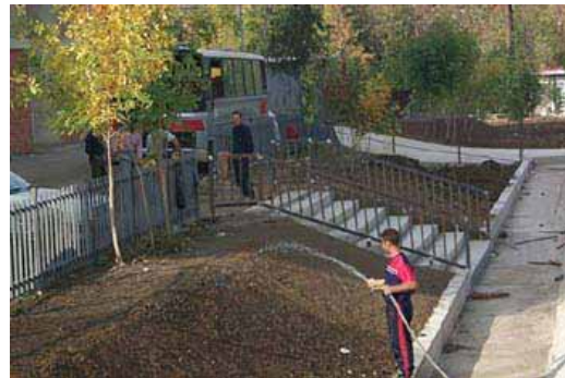
The land was cleaned, sculpted, planted; fences and stairs were installed.
