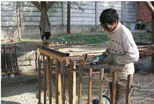
Welding and grinding the fences.
